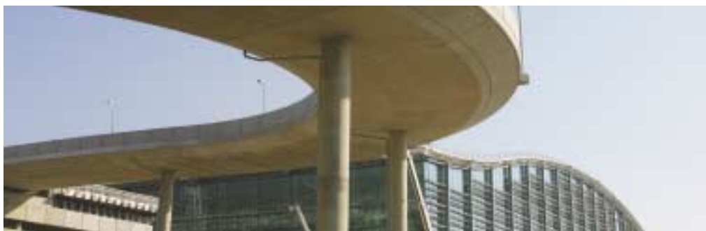
London Heathrow's new Terminal 5 (photo courtesy of BAA)
